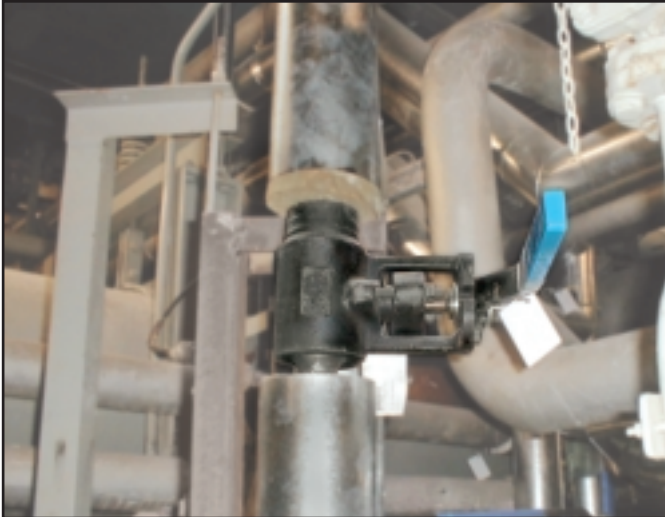
1 1/2" (40 mm) Power Ball Valves in steam trap isolation at a major British power plant. Switching to Velan Power Ball Valves offered a low torque, easy to operate solution.
